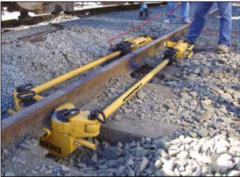
▼ RP70 Rail Puller in an obstructionless pull.
