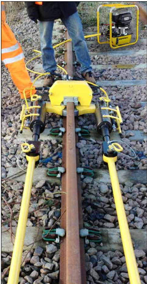
▼ The recommended power source for the RP70 is the Enerpac ZC-3404, for extreme force rail stressing.
