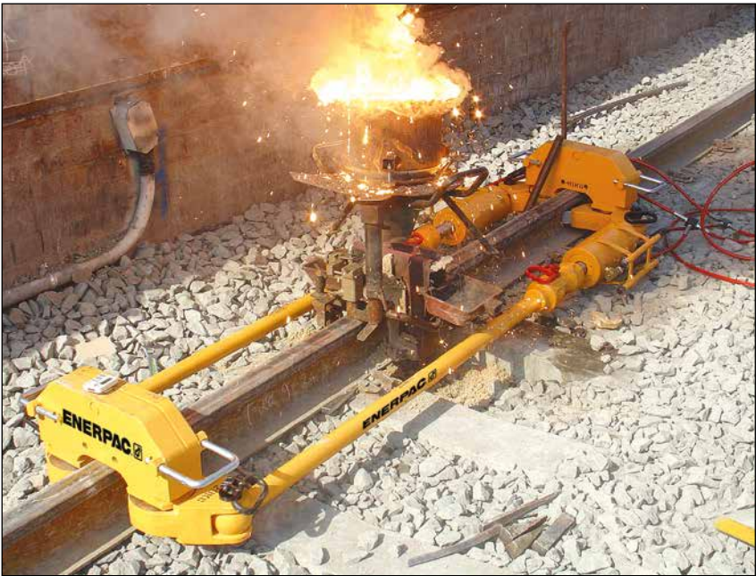
▼ RP70 Rail Puller in an obstructionless pull.
