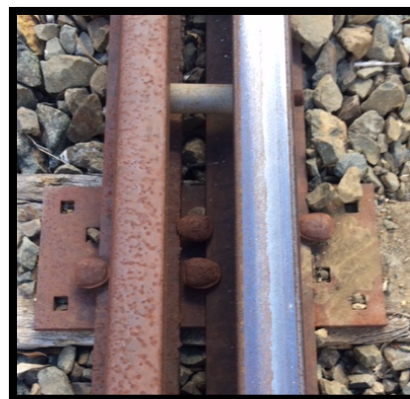
Pulls spikes between Check Rail
